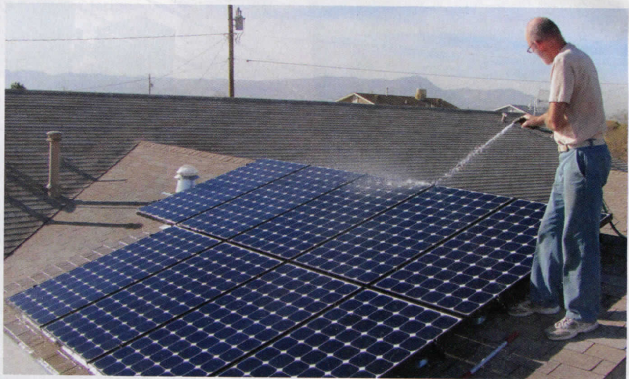
The system consists of nine 215-watt photovoltaic modules rated at 1.935 kilowatts.
